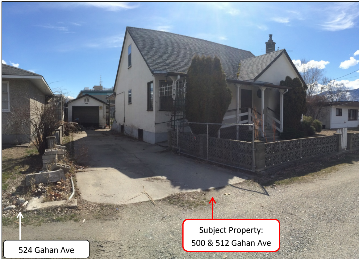
Figure 4 – Looking toward front of 500 & 512 Gahan Avenue from Gahan Avenue
