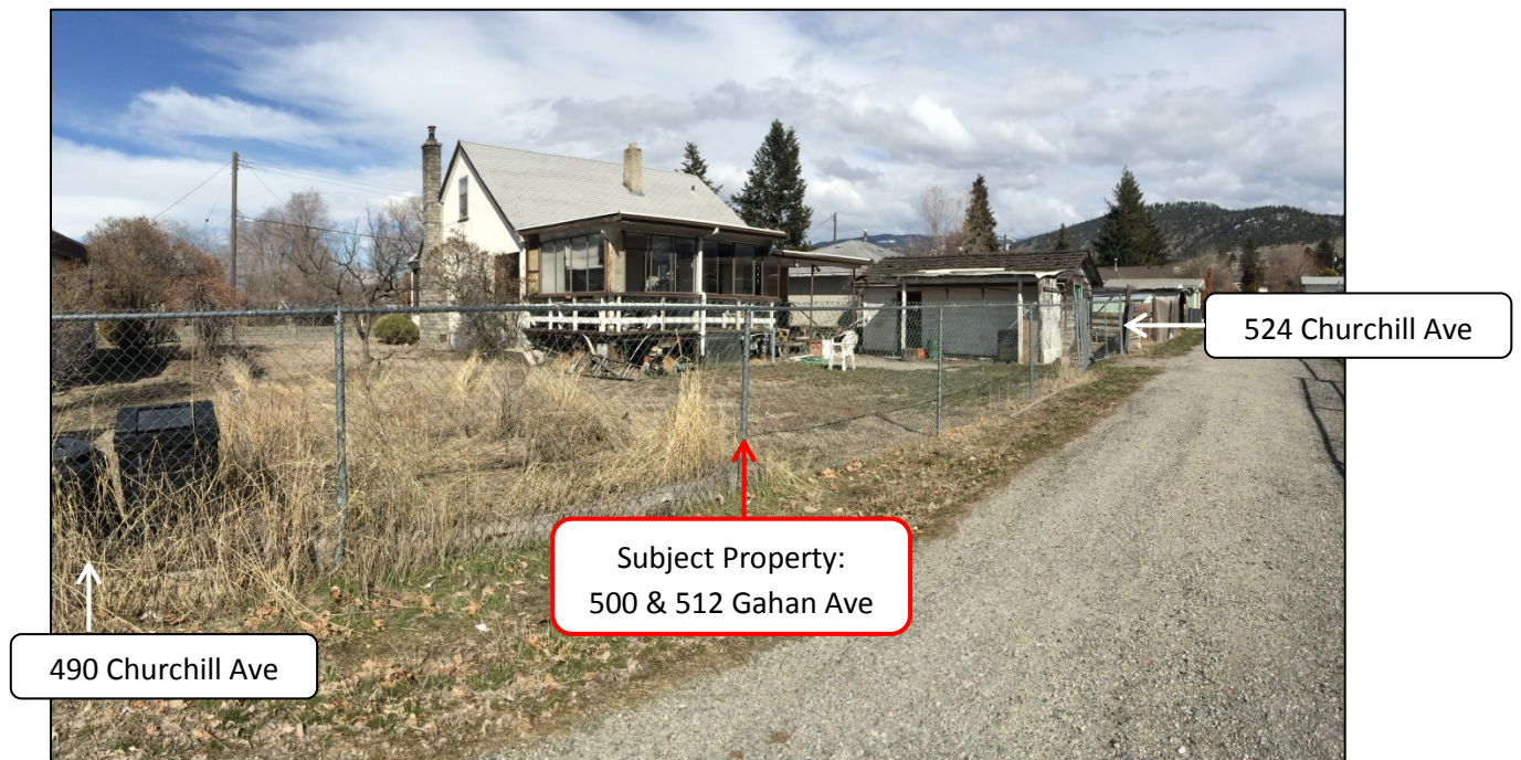
Figure 8 – Looking at 500 & 512 Gahan Avenue from the lane
