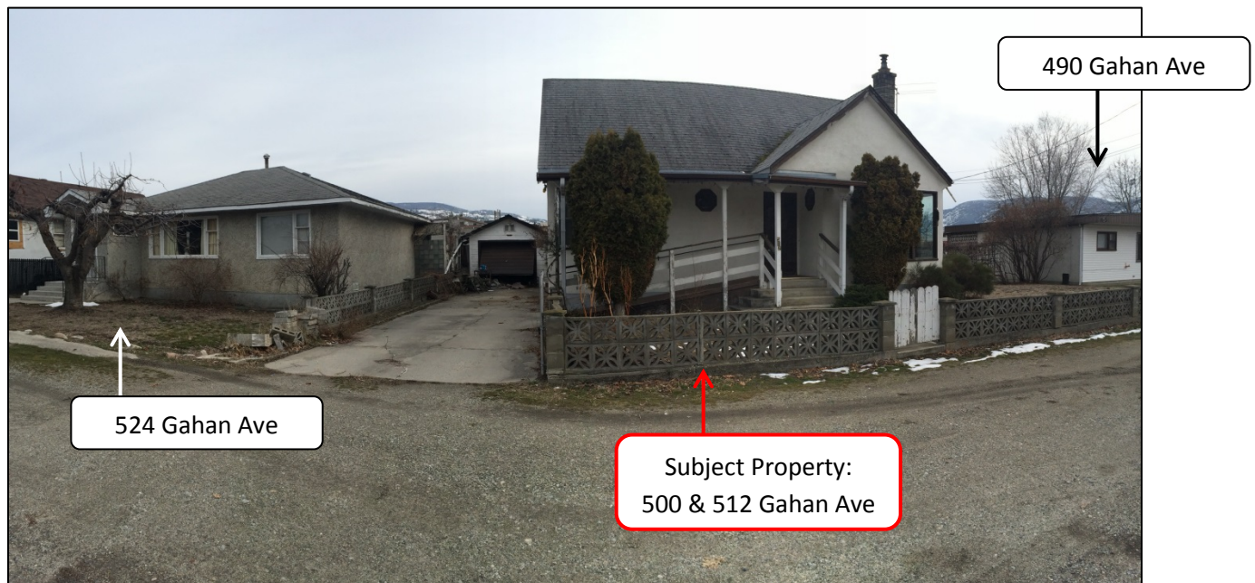
Figure 5 – Looking toward front of 500 & 512 Gahan Avenue from Gahan Avenue
